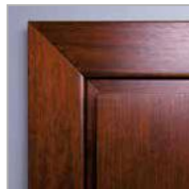
interconnection of architraves at an angle of 45°
